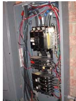
Electric panel door not replace after maintenance
