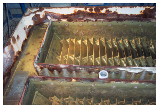
*Inclined Plate Clarifier in Plant 2 waste treatment.
