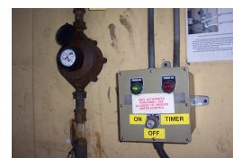
*Cycling switch and water meter.
